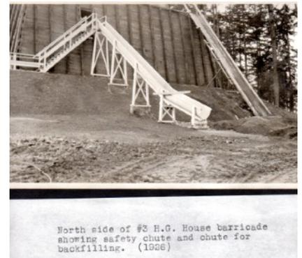
North side of #3 H.O. House barricade showing safety chute and chute for backfilling. (1926)
